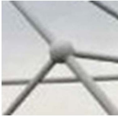
Fig. 4. Photograph of a typical node ball in a structure
