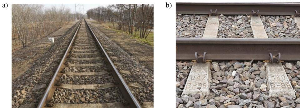
Fig. 1. Test section selected for TDR tests: a) view along the section; b) closer view of the ballasted track structure
