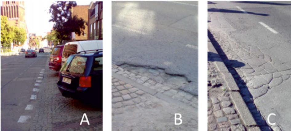
Fig. 2. Cycle lane Rajska–Podmłyńska: a) side parking b) uneven surface c) cracked surface
